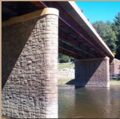
#904 Arroyo Bridge over Clarion River Elk County, PA
