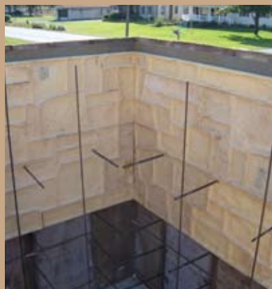
#898 Form Liner Installation
