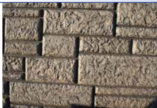
#908 BQE Old Cut Ashlar Stone
